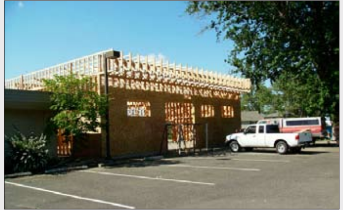
The new Sonbridge warehouse is almost complete.
