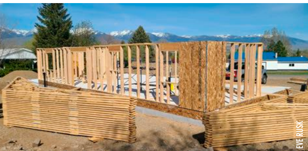
The church members have been busy building trusses.
