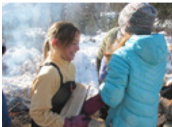
Tappahannock Junior Academy students help clear the site for the new cabin.
