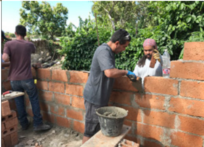
Ben Rodriguez (center) and Nathan McGee (right) lay bricks.
